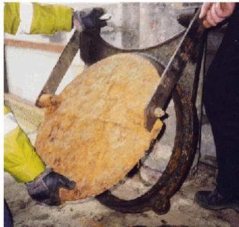
Figure 3. Steel flap valve used at downstream end of sluiced culverts. This flap gate has a seal of Ertalon Bush, and the edges of the circular gate fit flush into the steel ring surround, which is fixed to the concrete outlet structure.
