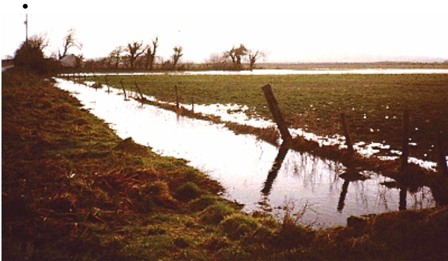
Figure 4. This back-drain is full and will shortly flood onto the surrounding field when fed from higher ground.
